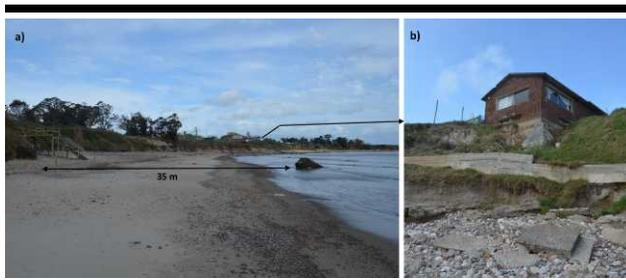
Figure 3. Evidence of cliff recession: a) 35 m linear distance was measured between old (concrete) and the new (wooden) cliff stairs; b) building at risk of collapse.
