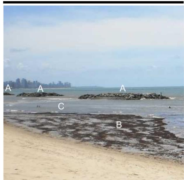
Figure 5. Breakwater configuration in a low spring tide (march 31, 2014) (A) three of the remaining breakwater sections, (B) a salience and (C) a bay formed by the wave-current sediment rearrangement just a few months after the breakwater reconfiguration.
