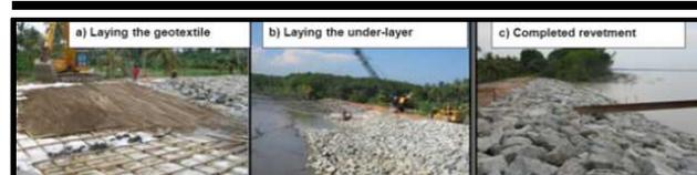
Figure 12. Activities during revetment construction: (a) laying of the geo-textile; (b) laying of the under-layer for the revetment; (c) completed revetment on the east coast of Tanjung Piai (DID Malaysia).
