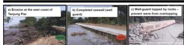
Figure 11. Erosion at the east coast of Tanjung Piai (a); completed seawall (well-guard) (b); well-guard topped by rocks to prevent from wave overtopping (DID Malaysia) (c).
